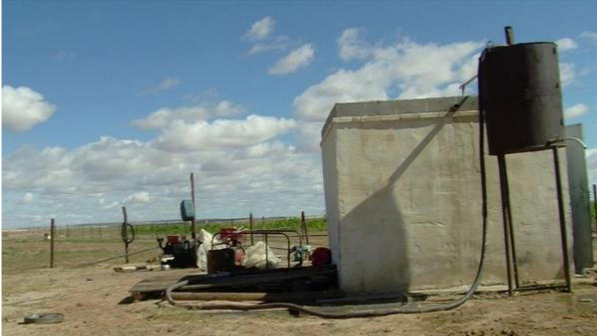
Figure 333: The new reservoir that Delgersaikhan has had installed at the farm. The well inside the building has been drilled to a depth of 80 metres, with the water surface located at 27 metres underground; this well provides one tonne of water per day.
